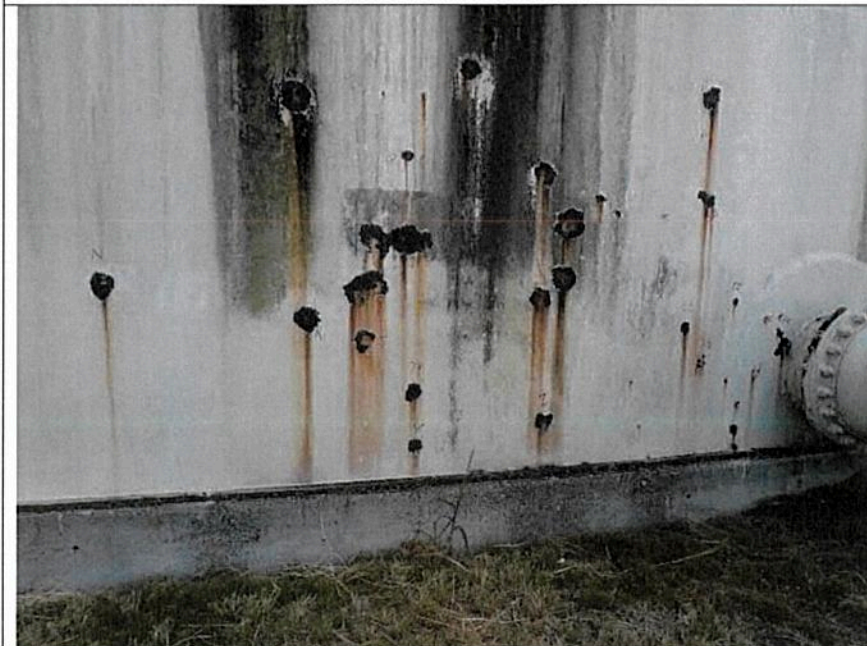
Localized corrosion on first shell course
