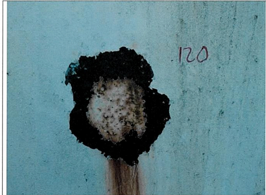
Localized shell corrosion
