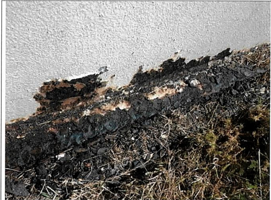
Corrosion on projection plate and chime area
