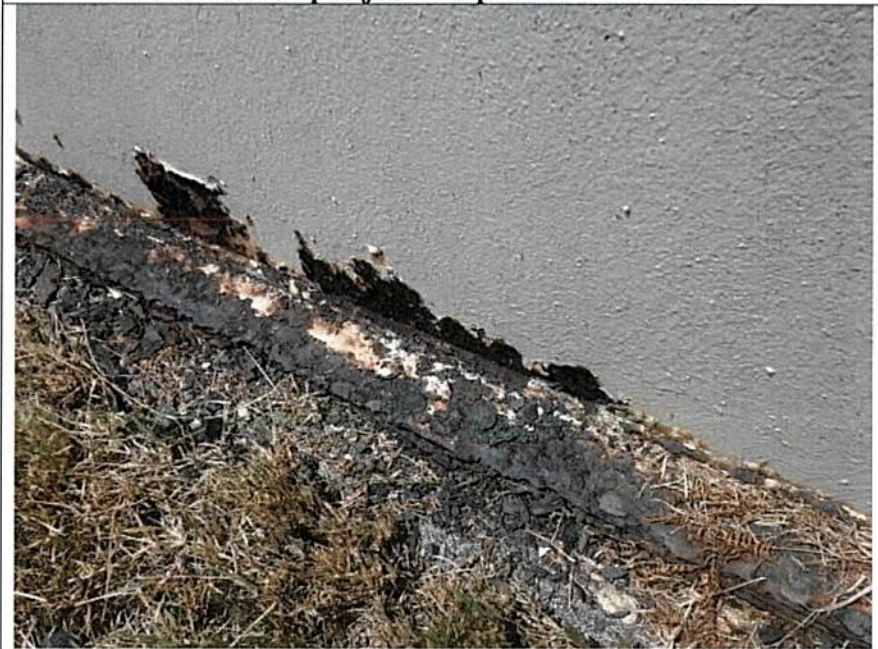
Corrosion on projection plate with knifing noted
