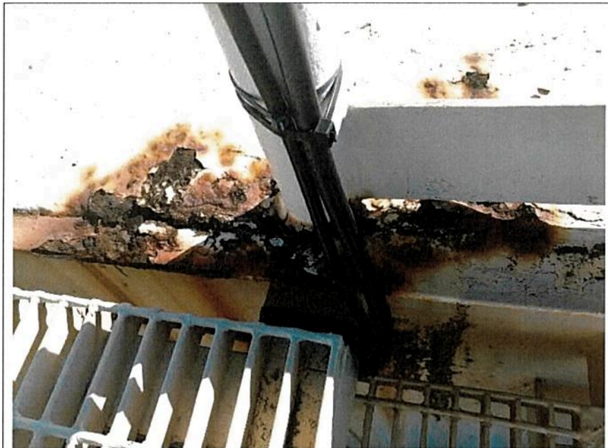
Corrosion at handrail support of tank roof
