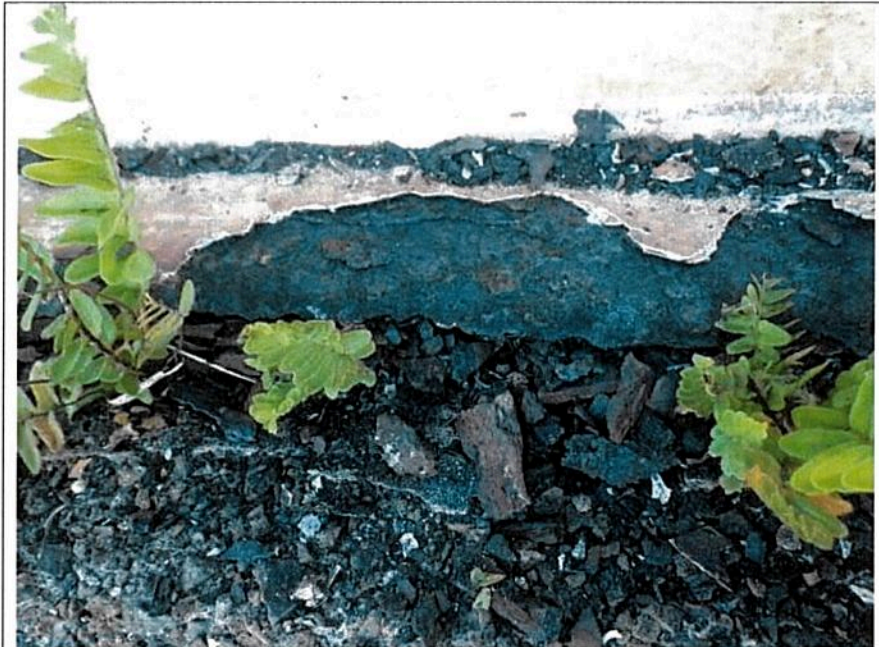
Knifing of the projection plate and vegetation growth
