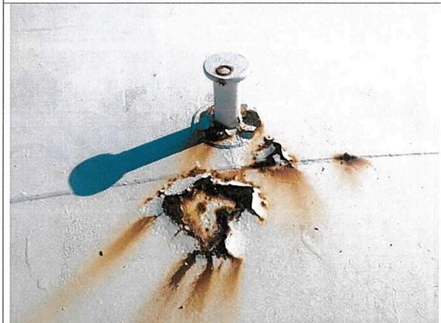
Scaffold ring with corrosion at reinforcing plate
