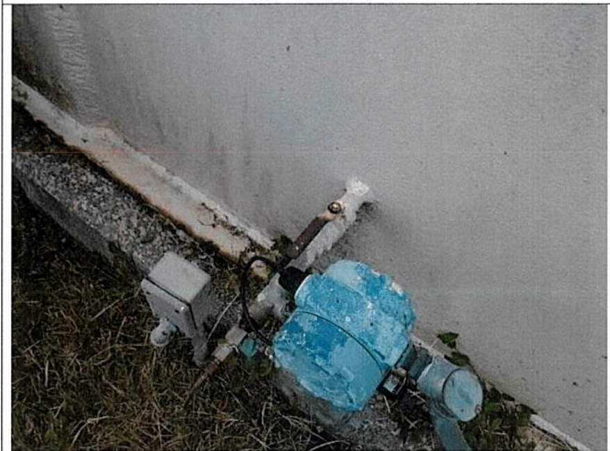
1" nozzle without seal weld to block valve
