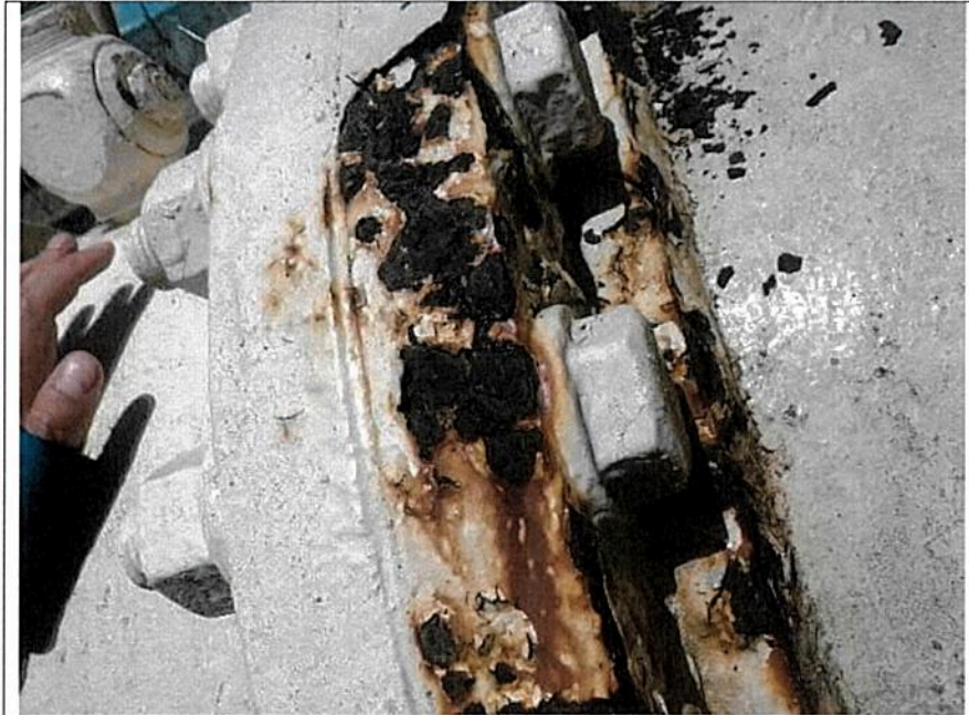
Flange corrosion on nozzle (typical)
