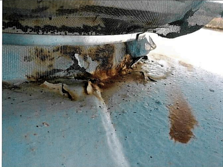
24" roof vent nozzle with corrosion on nozzle bore and attached mesh screen
