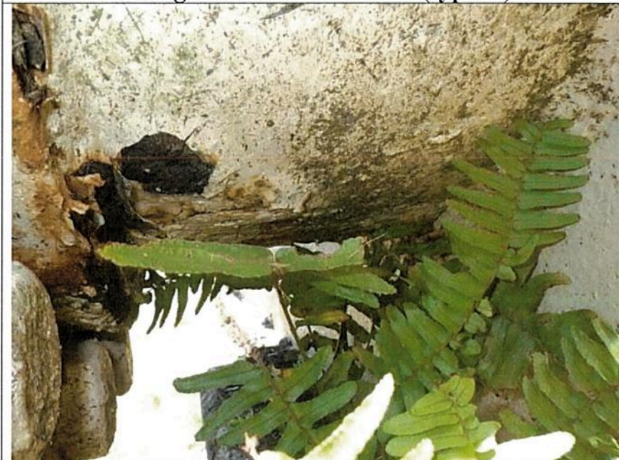
Vegetation growth around tank (typical)
