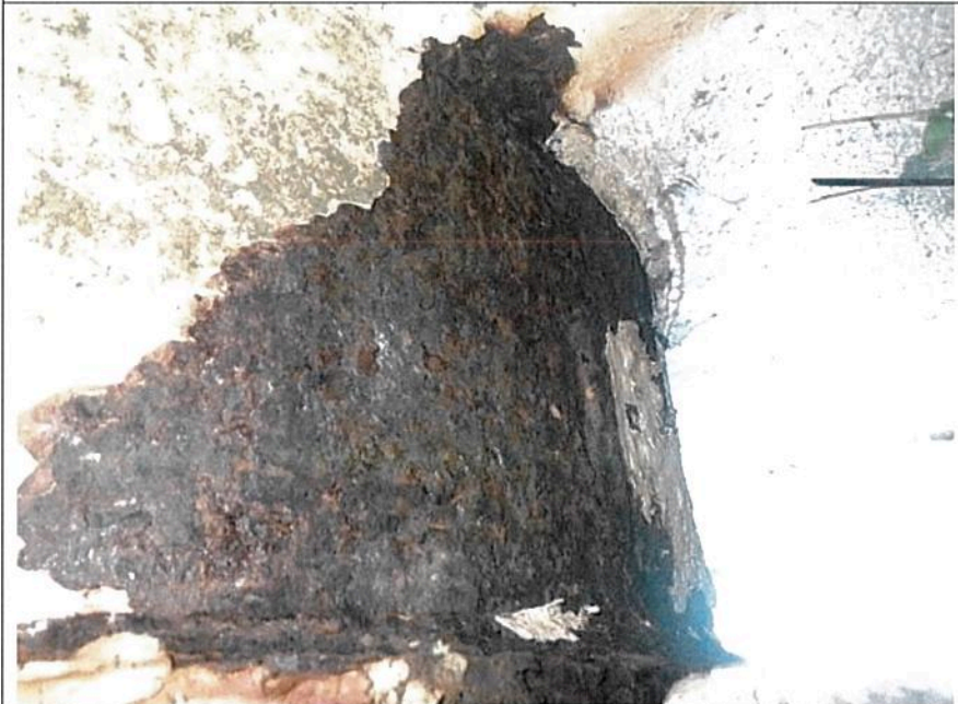
Underside corrosion of the Fill/Suction Nozzle
