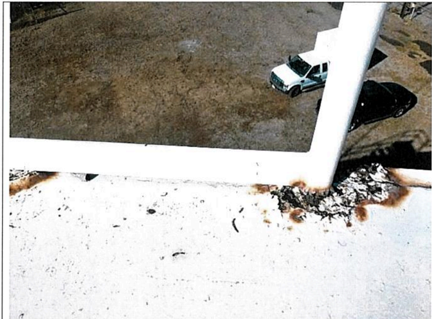
Corrosion at handrail support at peripheral edge of roof
