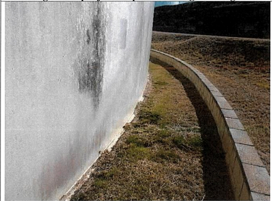
Vegetation growth along east side of tank projection plate
