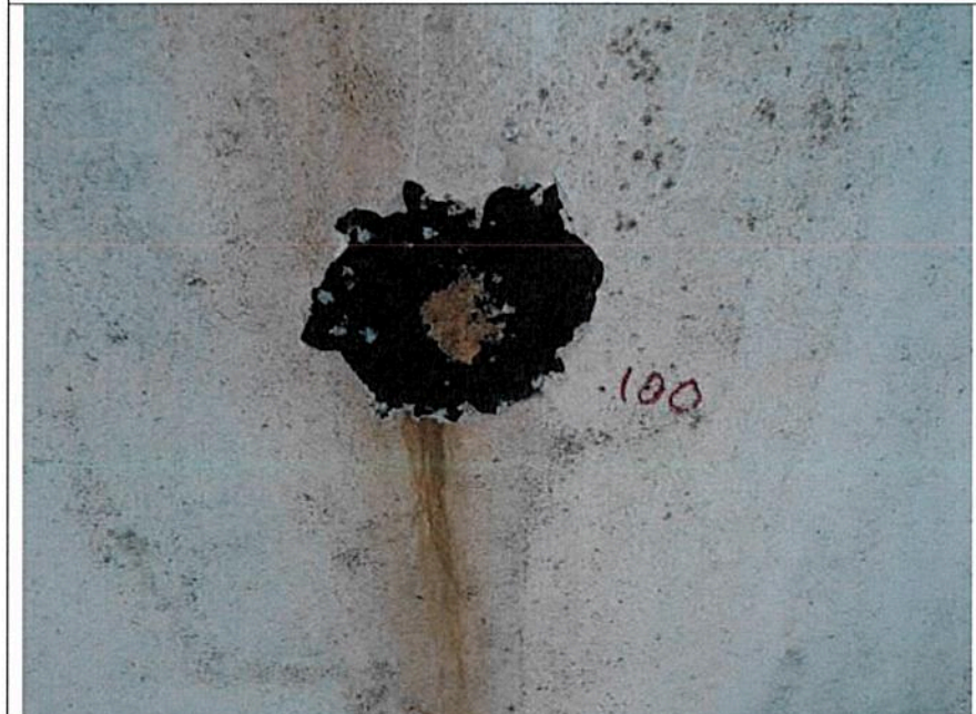
Localized shell corrosion
